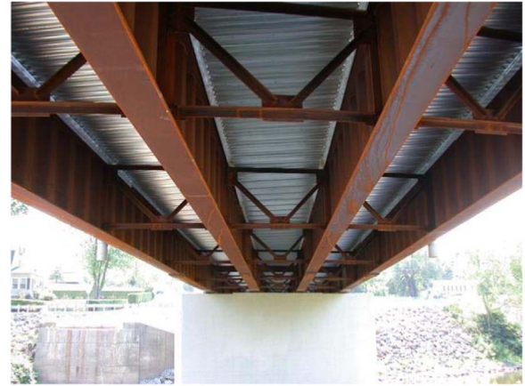
Fig. 2. HSS demonstration bridge with corrugated webs in Bradford County, USA [23].
