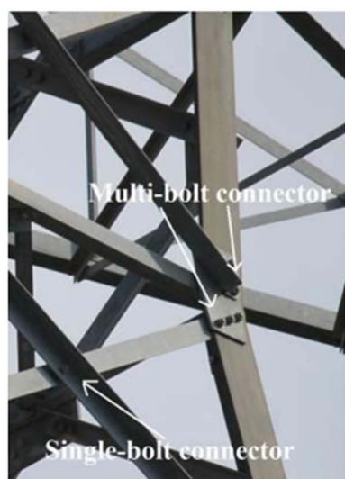
Fig. 1. Single/Multi-bolt connector.
