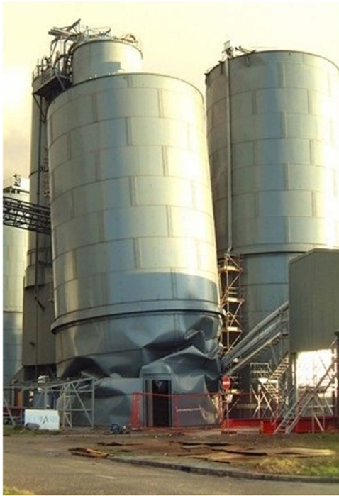
Fig. 1. A collapsed steel silo caused by axial compression.
