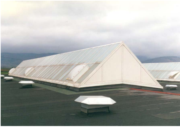
Fig. 1. Long skylights in industrial hall bay A–B between transverse systems 2–6.
