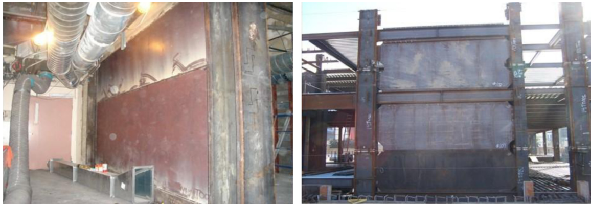
Fig. 1. Typical implementation of steel shear walls.
