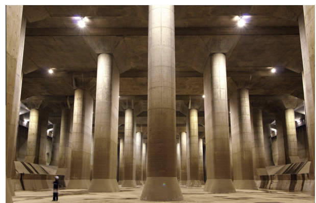
Fig. 2. Metropolitan area outer underground discharge channel. ( http://www.ktr.mlit.go.jp/edogawa/gaikaku/english/index.html ).
