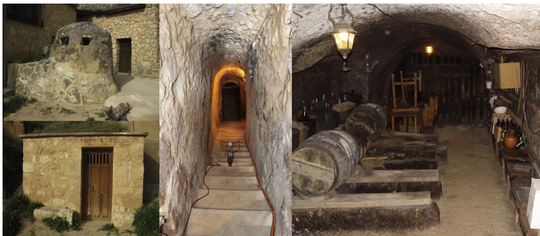
Fig. 1. Detail of the entrance, ventilation chimney, access tunnel and cave to the construction analyzed.
