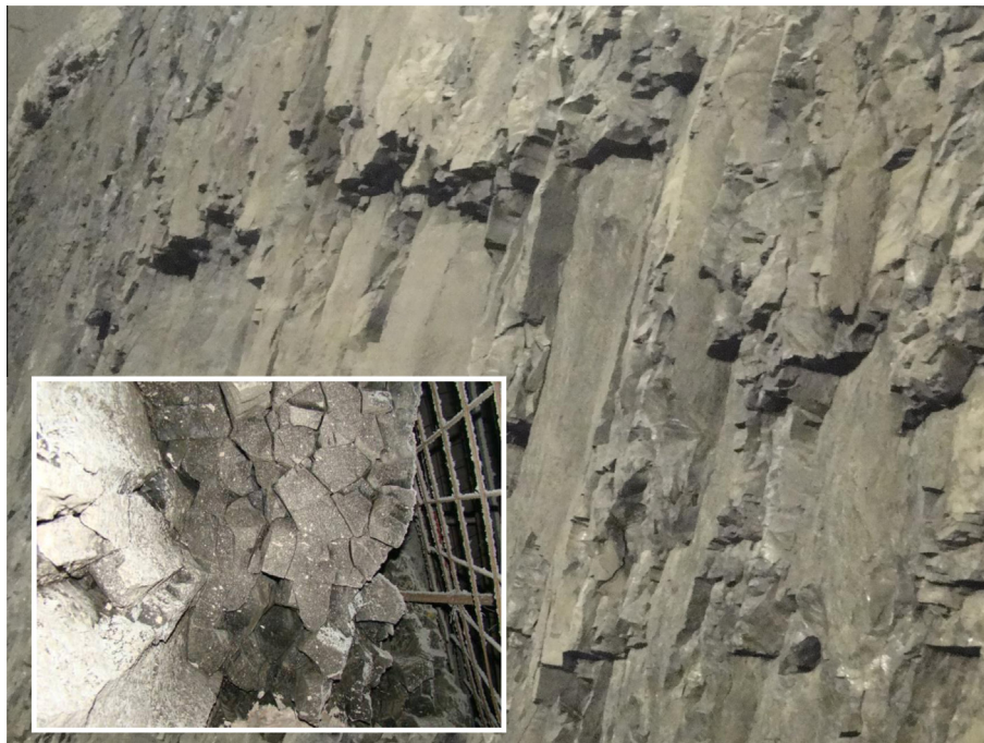
Fig. 1. Steeply inclined columnar joints oriented normal to a breccia plane. In the inset a cross section through the lava flow shows the polygonal geometry of the columns (see Jiang et al., 2014).
