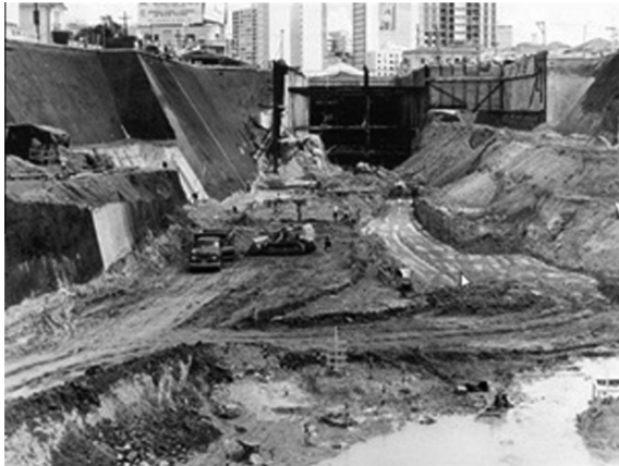
Fig. 1. Deep bench excavation.
