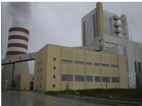
Fig. 1. Electric power plant of Meliti.
