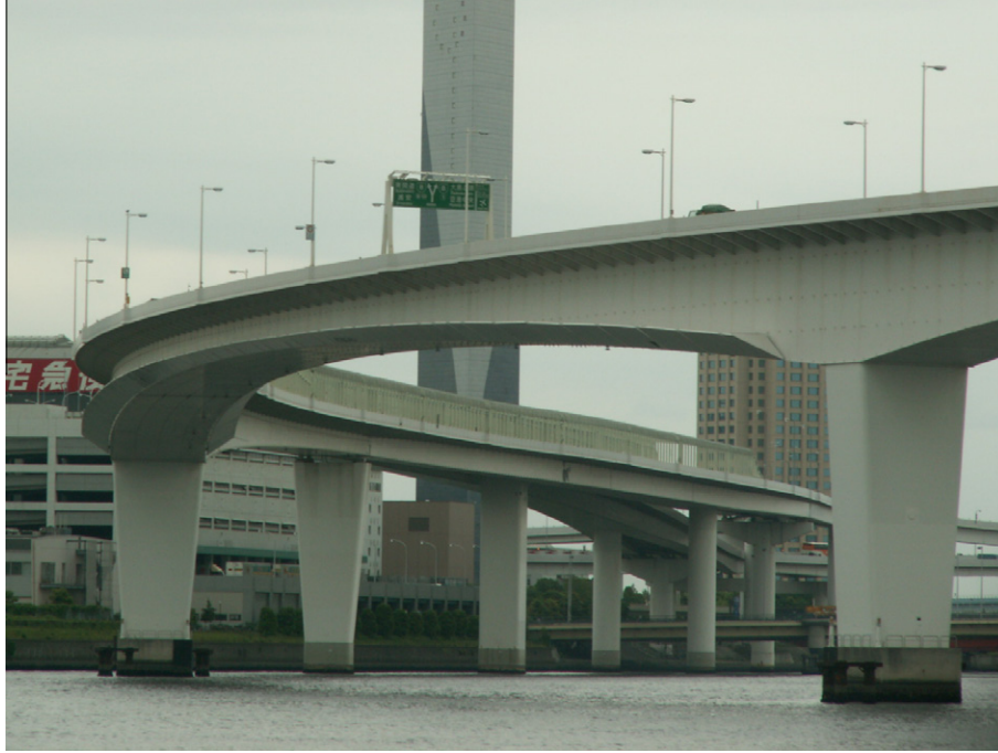
Fig. 1. Metropolitan Expressway Route 11 Daiba line.
