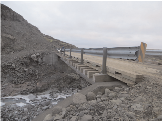
Fig. 2. Bridge where camera was installed. Circle marks camera position.
