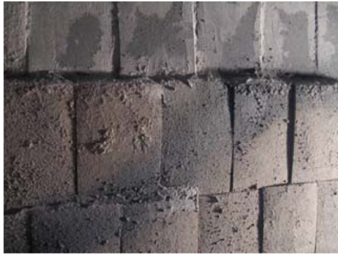
Fig. 1. New (top) and old (bottom) SiC-based refractory tiles in a WTE facility; picture taken about 7 m from the burning grill after a long period of plant operation (tile height: 245 mm).
