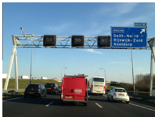
Fig. 1. VSL implementation on A13. Delft, The Netherlands.
