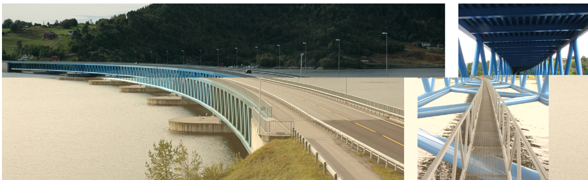
Fig. 1. Left: The Bergsøysund bridge viewed from the northeast end; right: the truss structure as viewed from below the bridge deck. Photo: K.A. kvåle.
