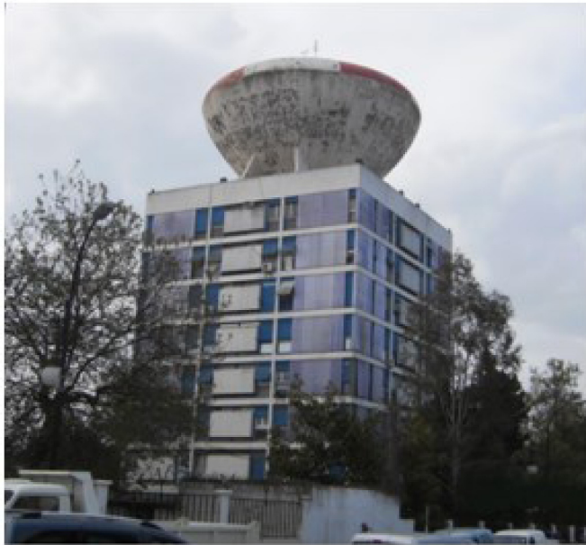
Fig. 1. General view of the structure (building-tank).
