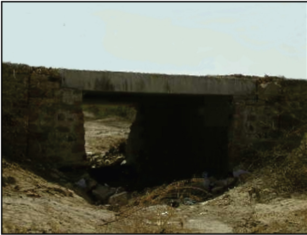
Fig. 1. Reinforced concrete slab bridge.
