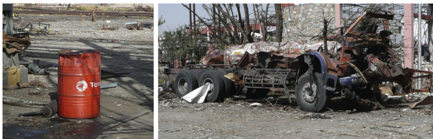
Fig. 1. Pressure Damage at Jaipur.
