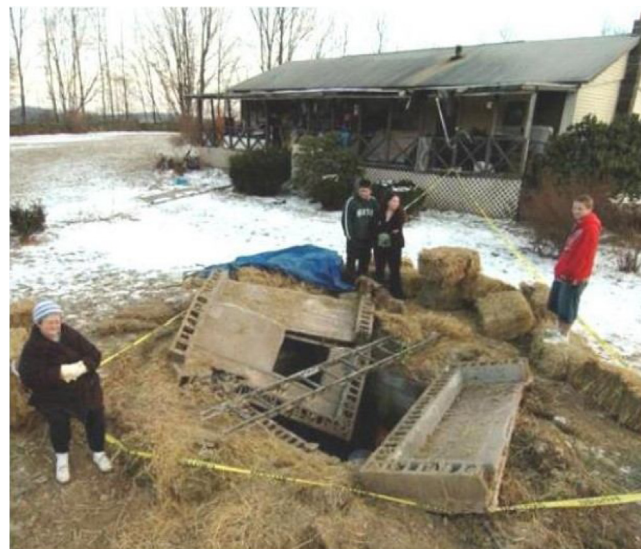
Fig. 2. Dimock water well vault and the two sections of the split and overturned concrete slab with the top course of concrete blocks still attached. View looking to the southeast. A reporter from the Scranton Times-Tribune appeared with a photographer the morning after the event in question (Legere, 2009). The reporter believes that the broken concrete slab had not been moved between the time of the January 1st 'explosion' and the time of this photograph was taken less than 24 h later (L. Legere, 2013, personal communication).
