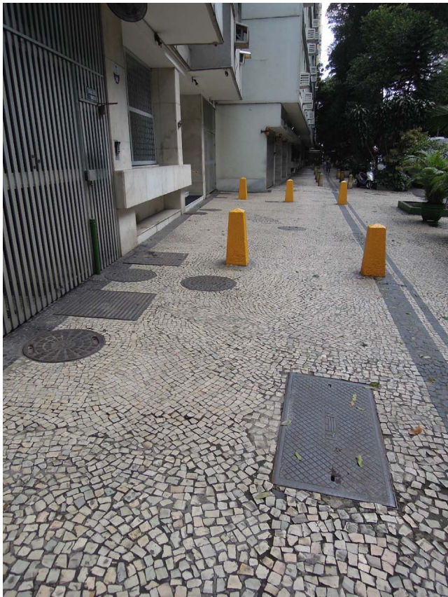
Fig. 1. The subsurface infrastructure. This street scene in Rio de Janeiro, Brazil illustrates the many types of covers that provide access to subsurface structures. The access cover provides little if any information about what lies underneath.
