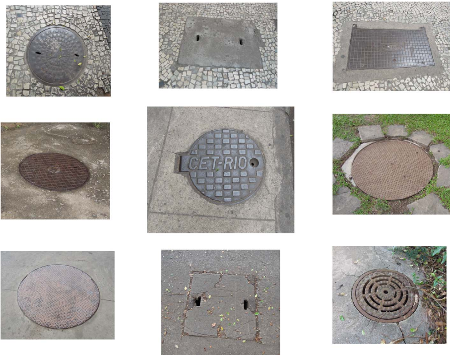
Fig. 2. Access covers on subsurface structures. Access covers include cast steel manhole covers, extruded aluminum hatches, steel plates, and poured concrete hatches.
