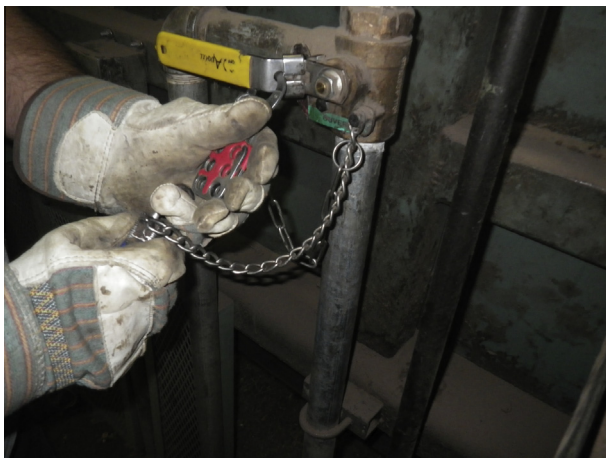
Fig. 1. Application of a padlock during a lockout procedure.
