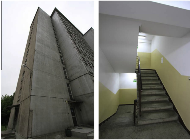
Fig. 1. Building and the staircase.
