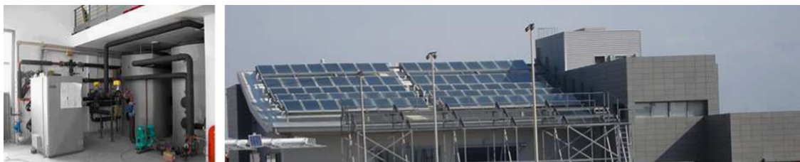
Fig. 1. The CIESOL building (Camacho et al., 2012) showing two pictures corresponding to the accumulation tanks and solar collector field.
