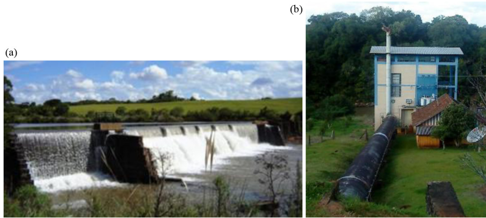
Fig. 1. Small Hydropower Plant's reservoir, penstock and housing.
