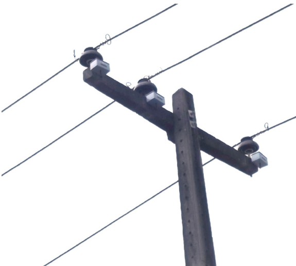
Fig. 2. A set of three sensors installed in a power line structure.
