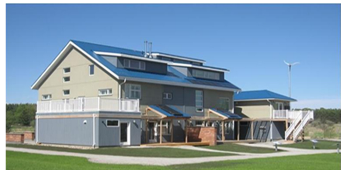
Fig. 1. South-west side of twin houses at Toronto and Region Conservation Authority (TRCA).
