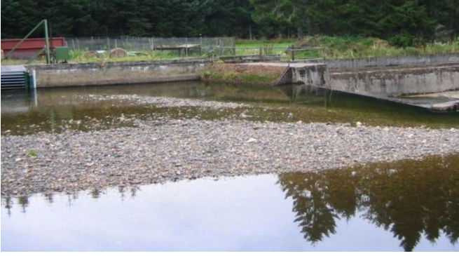
Fig. 1. Sediment upstream weir.
