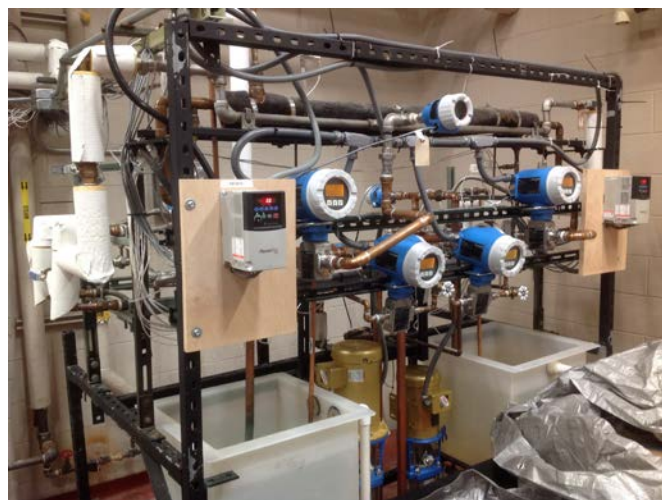
Fig. 2 Shell-and-tube heat exchanger experimental area.
