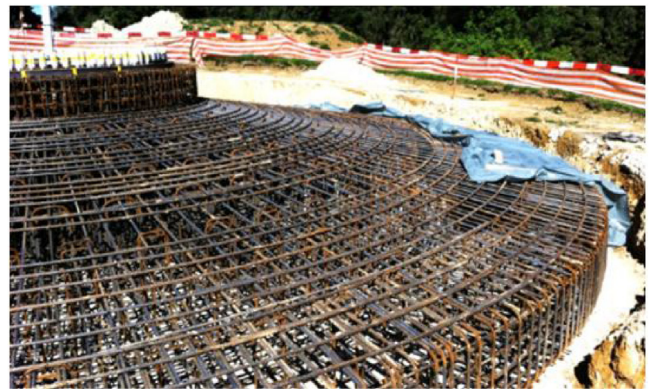
Fig. 3. Grounding system of WT6.
