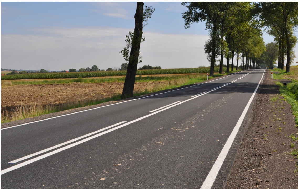
Fig. 1. Mud and soil on a porous pavement brought from fields by agricultural vehicles (photo by M. Motylewicz).
