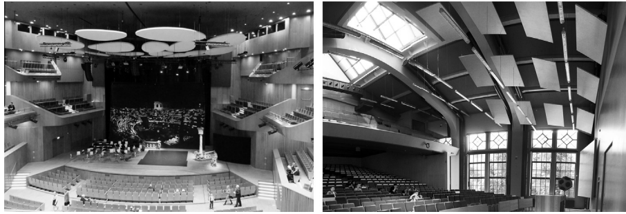
Fig. 1. Reflective panels suspended over the stage in ICE Congress Center, Cracow (on the left) and in AGH conference hall, Cracow (on the right).
