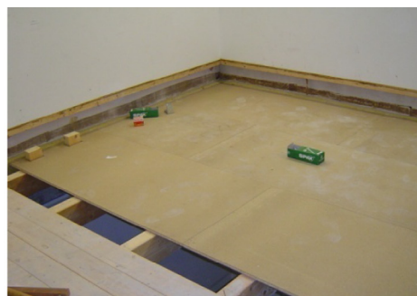
Fig. 1. Left, fan unit, free-standing in laboratory area, with two of the four contact points indicated; Right, timber joist chipboard floor under construction.
