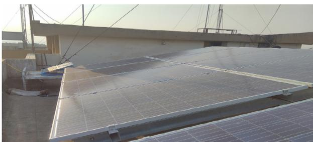
Fig. 1. A section of a PV plant getting shaded every day during evening hours due to neighboring structures.
