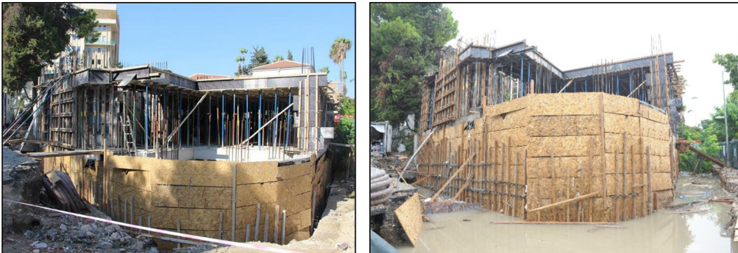
Fig. 3. Photographs of the examined structure before and after the floating.
