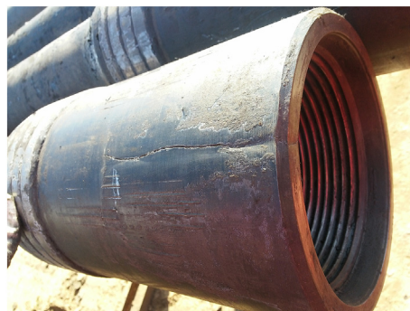
Fig. 1. Outward appearance of the failure joint of drill pipe in the field.
