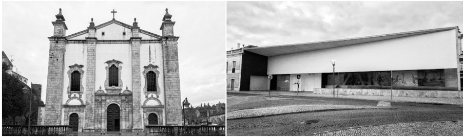
Fig. 1. Example of an historic building with various protrusions intended to protect the façade from the water flow (left) and a contemporary building with a single protrusion that is effective in protecting the façade from humidity-related issues (right).
