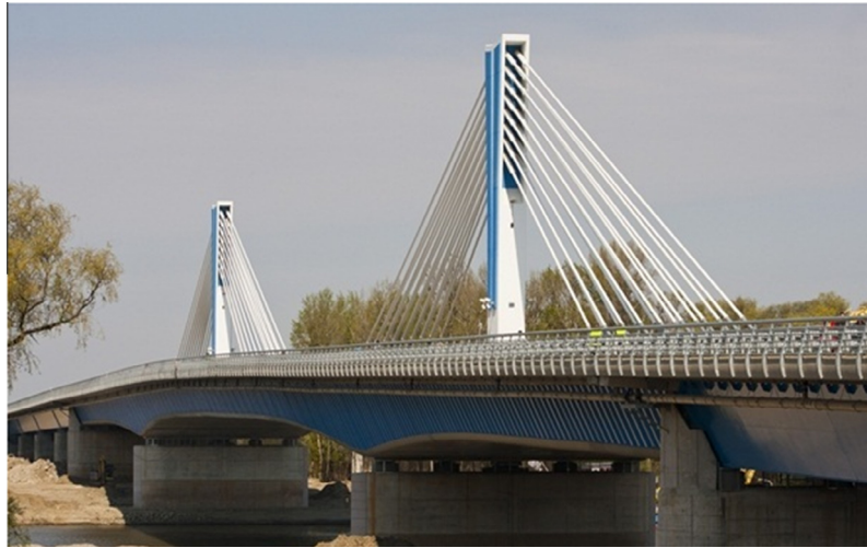
Fig. 1. Móra Ferenc M43 highway bridge on the Tisza river [2].
