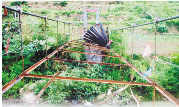
Fig. 1. A footbridge after ATD.
