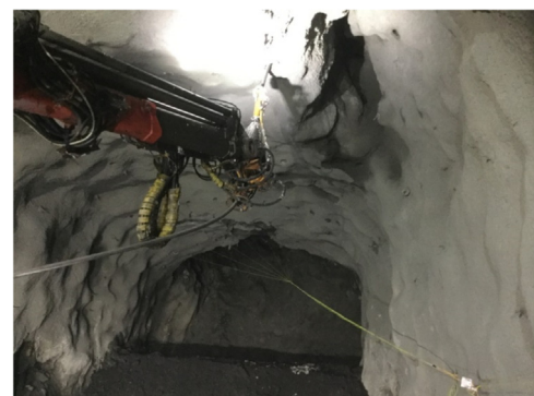
Fig. 2. Observation of charging procedure in a borehole.
