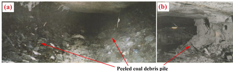
Fig. 2. The distribution of peeled coal debris piles in coal mines, U.S. 11 : (a) peeled coal debris piled around pillar in Hiawatha 2 seam; (b) peeled coal debris piled around pillar in Hiawatha 1 seam.
