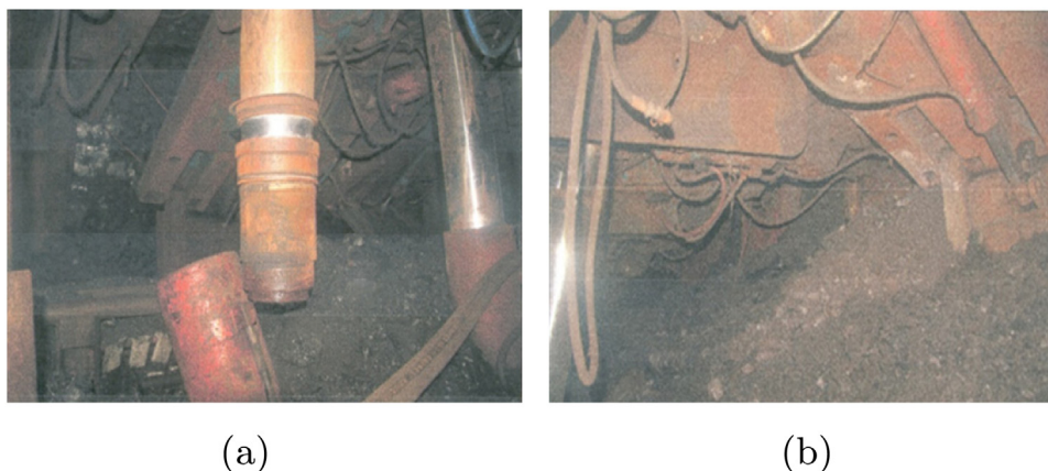
Fig. 2. Photographs of an OII rockburst in LW3112 at Chaoyang Coal Mine showing (a) collapsed supports and (b) blocked gate roads.
