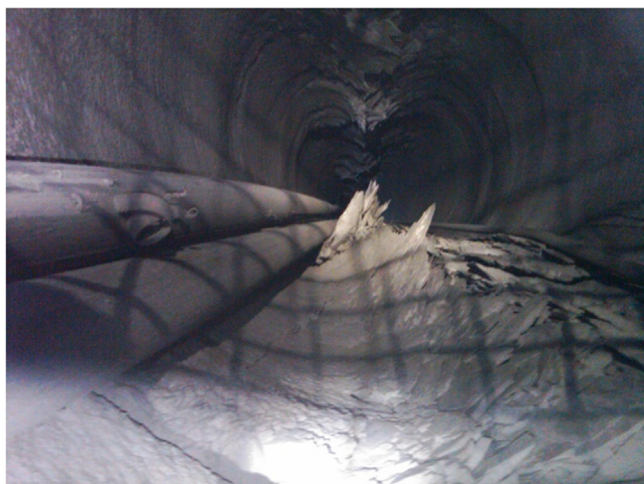
Fig. 2. Example of stress-induced argillite buckling in a raise at the Lucky Friday mine (after 4 ).
