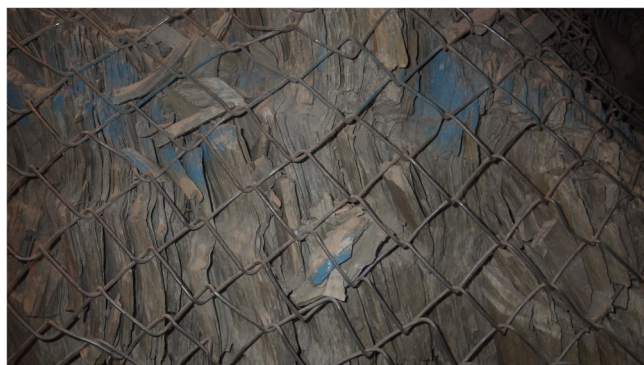
Fig. 1. Photo from the Lucky Friday mine showing the argillite unit through which the #4 shaft was excavated; the kinking of the beds shown in this photo is present in some locations, but is not ubiquitous throughout the unit.
