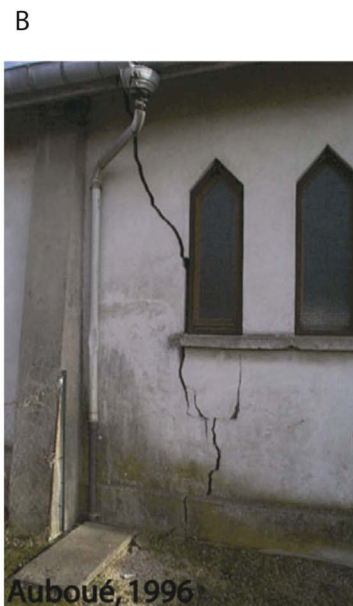
Fig. 2. Description of the main characteristics involved in mining subsidence and their associated consequences. (A) Typical profiles of the ground displacements. (B) Example damage due to mining in the city of Auboué in 1996, France.
