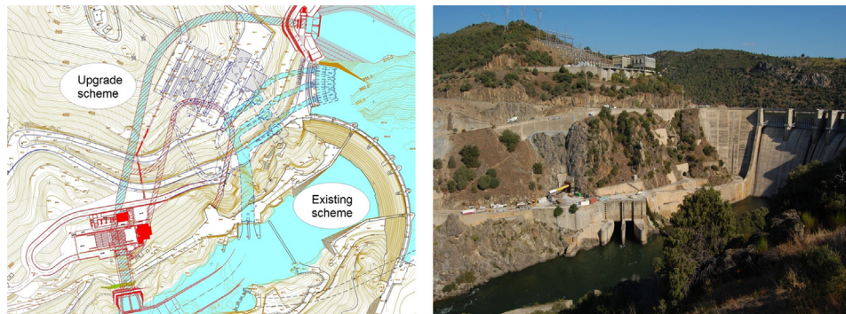
Fig. 1. Map of the surface, hydraulic circuit, powerhouse and auxiliary adits. (left), adapted from [11]. Photo of the dam and right bank during construction of the upgrade (right).
