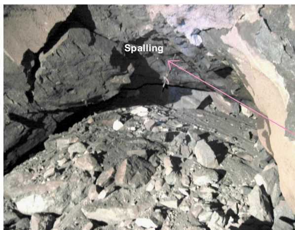
Fig. 2. Dynamic rock fracture—spalling—close to explosive charge when a primer is located near the collar. The shadow area is the region occupied by tensile stress waves when one portion of explosive in the boreholes is detonated.
