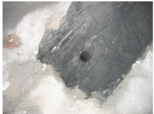
Fig. 4. Dynamic fracture—spalling—in the free surface (drift wall) due to the single shot. The volume of the broken region is about 1 \text{ m} \times 1.2 \text{ m} \times 0.2 \text{ m} .
