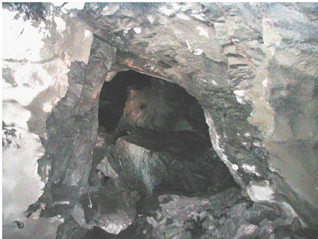
Fig. 1. Church-shape drift roof due to blasting [1].
