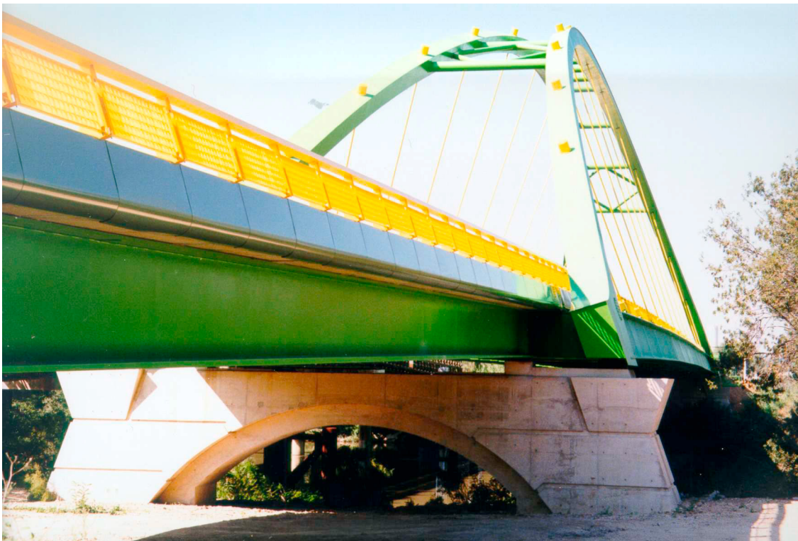
Figure 1 : Saint-Gilles bridge crossing the Rhône
