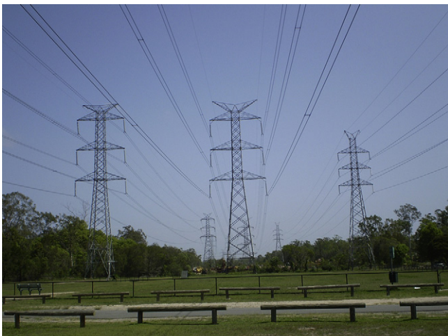
Fig. 1. The measurement site showing the three sets of double circuit lines.
