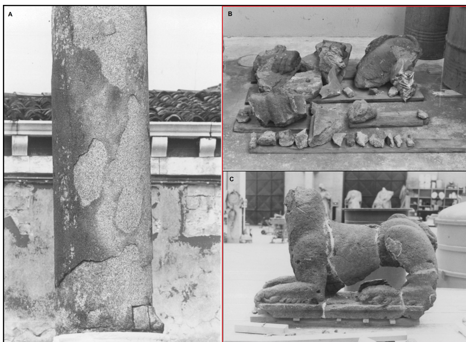
Fig. 1. State of conservation of an ancient Mysian granite column on the Island of Murano before consolidation treatment (A) and the trakyte Gatta di Sant'Andrea in Padua before (B) and after (C) restoration using EP2101.
