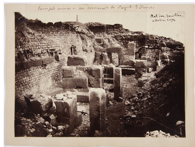
Fig. 2. Ruins of the temple of Mercury atop Puy de Dôme volcano. All white building stones are made of the same trachyte (photograph dated 1874, Archives Départementales du Puy-de-Dôme, 154Fi-13).
