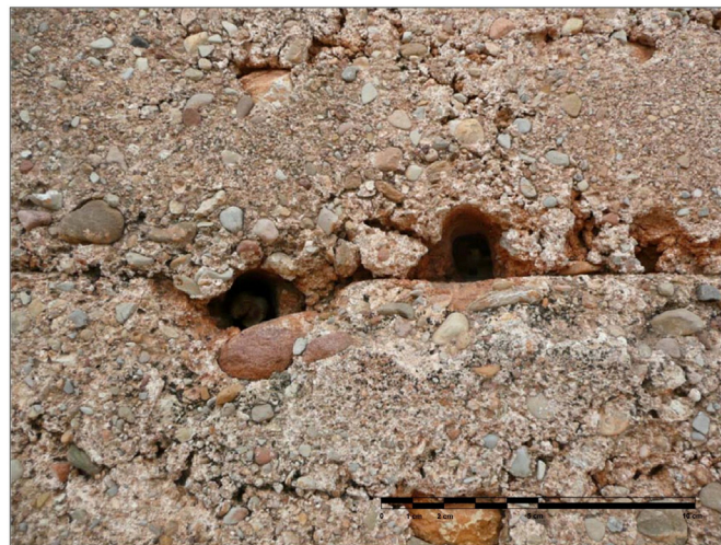
Fig. 3. Putlogs of the formwork inside the walls of Bofilla Tower (C. Mileto and F. Vegas).
